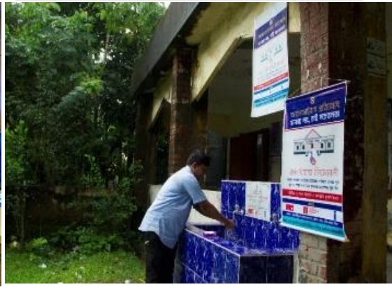
Installation of handwashing facility at UP level by EALG project
